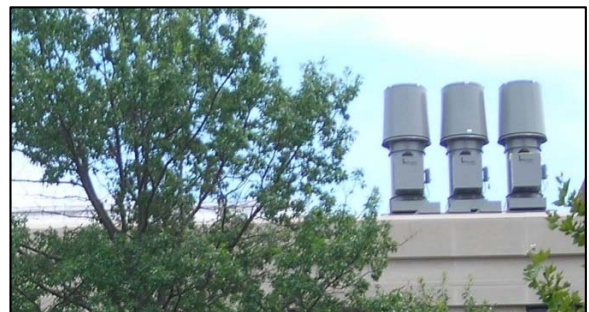
the three exhaust outlets
