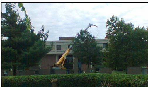
the big crane lifting material to the roof
